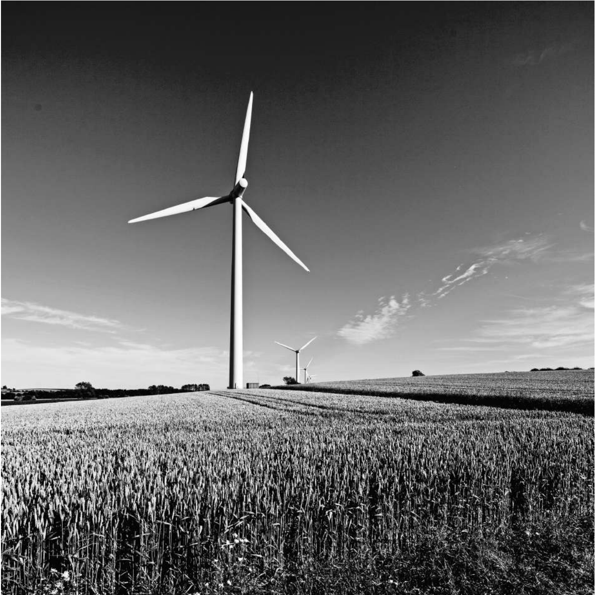
Denmark helped lead the way on making wind power more affordable. These turbines are on the island of Samsø.
