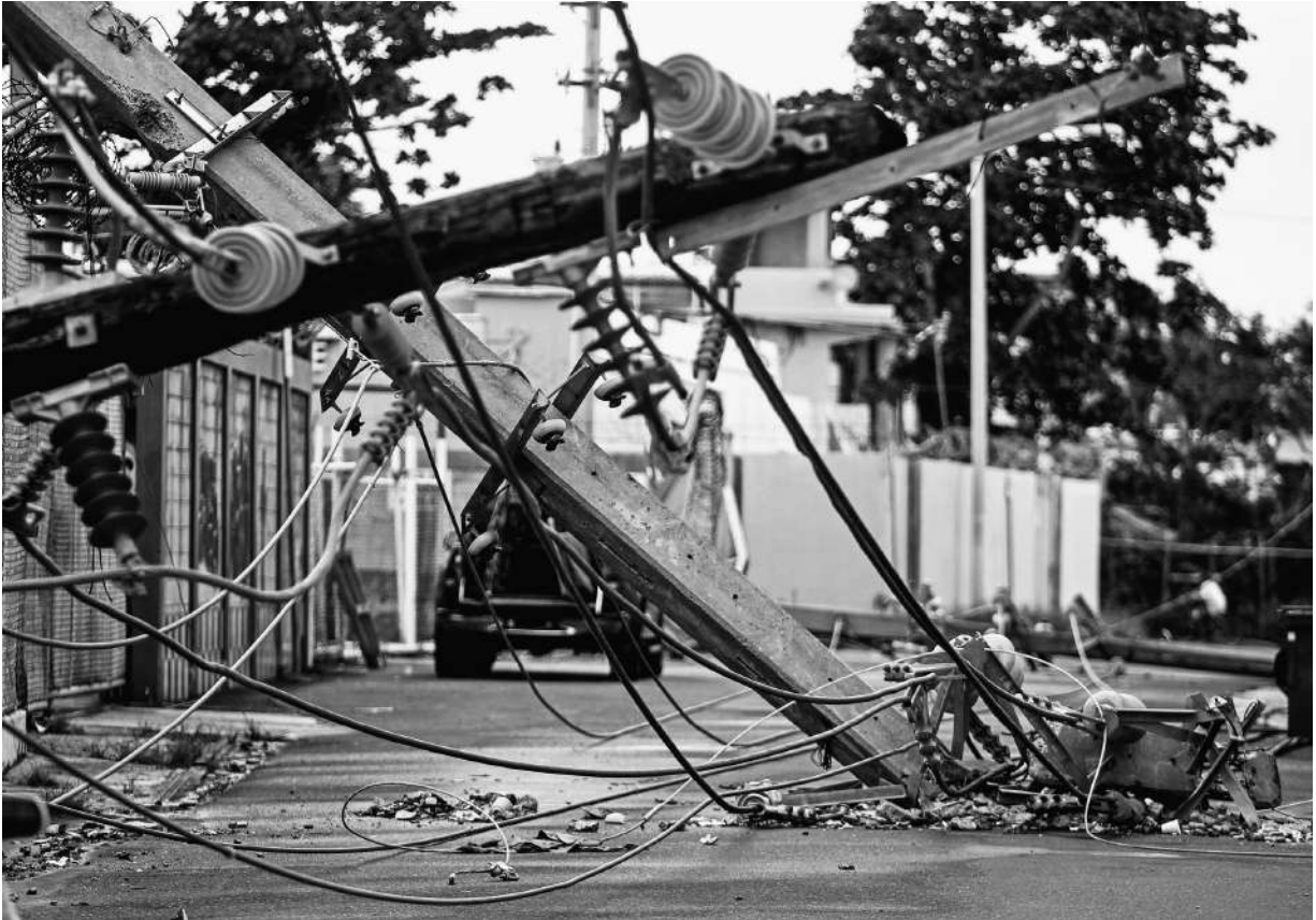
Hurricane Maria set Puerto Rico's power grid and other infrastructure back some two decades, according to one study.
